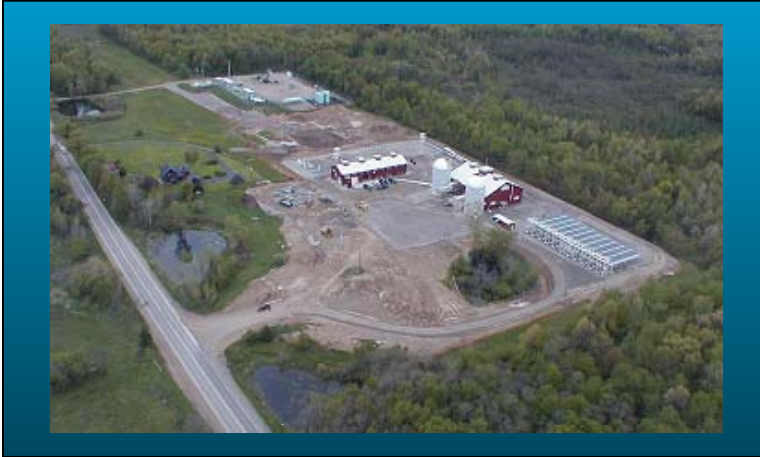
Figure 6: Compressor Station Site
